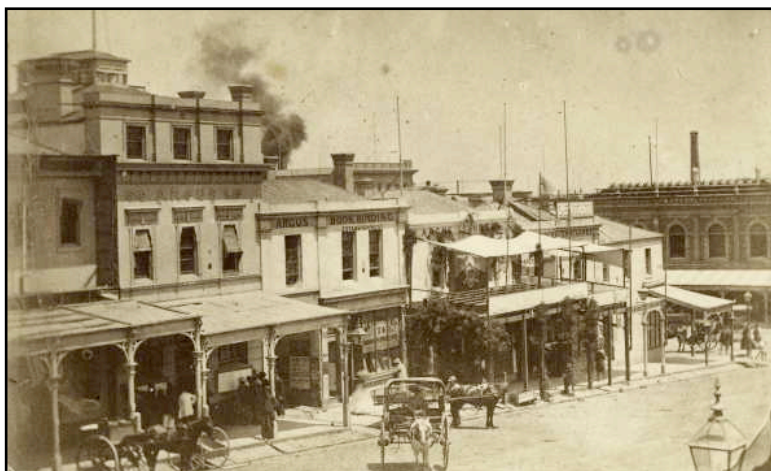
Above: Argus Office, 76 Collins Street East, Melbourne,
